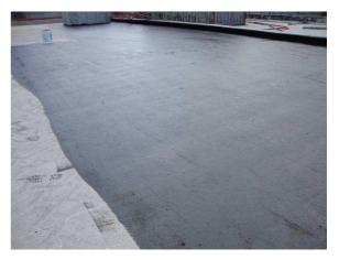
Substrates that are very dry and absorbent must be dampened before application to ensure good adherence. The product must not be applied in the rain.
