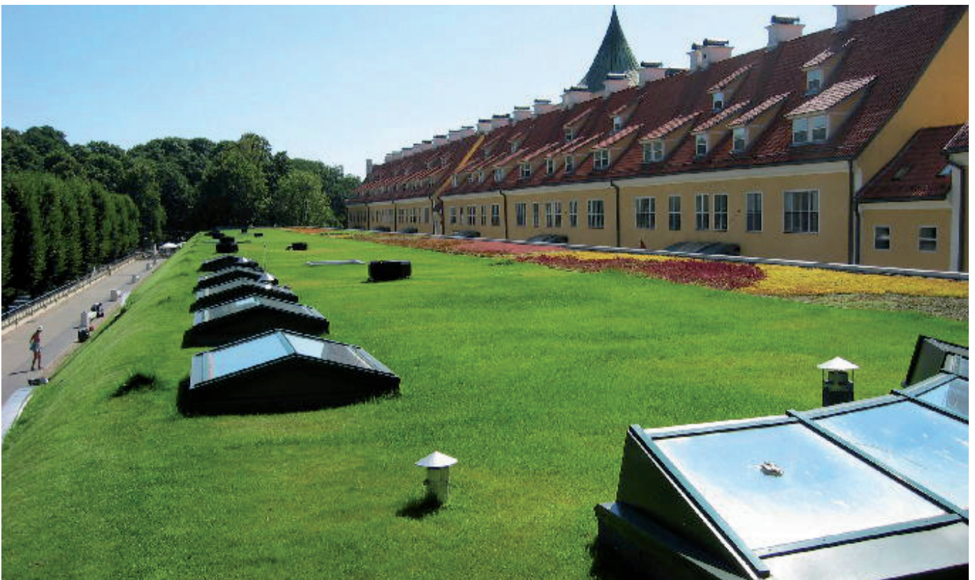
Parking enterré - Riga - Lettonie
