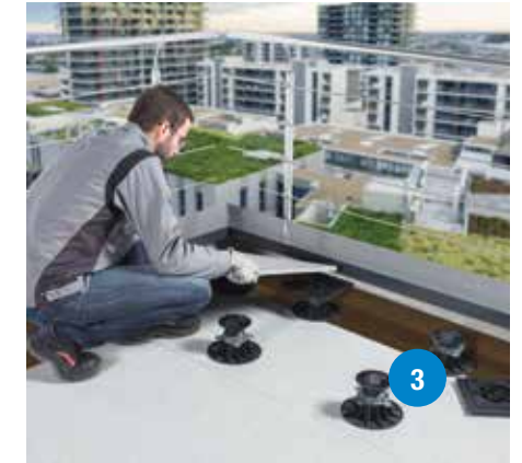
Place the first slab forming the patio corner and adjust it.
