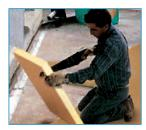
1. Cutting and installation of the insulation loose and in staggered pieces
