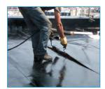
3. Heat welding the overlaps of the 1st layer of waterproofing
