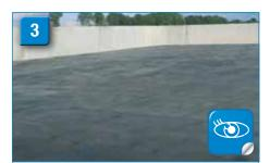
Do not wet the surface until product is not completely dry. Product must be dry before applying waterproofing membranes.
