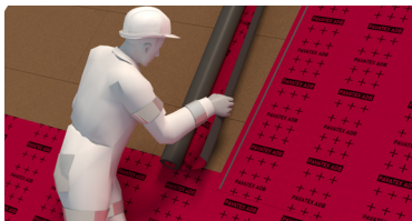
Sealing lateral overlaps with PAVATAPE 12 (ABD membrane).
