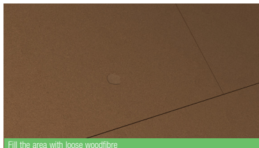
Fill the area with loose woodfibre
