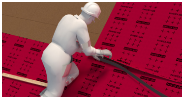
Self-sealing longitudinal overlaps (ABD membrane).
