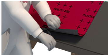
Best practice is to seal the membrane on the eaves tray to avoid snow water back pressure. PAVATAPE 12 (ADB membrane)
